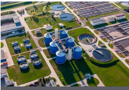
Sewage treatment plants
