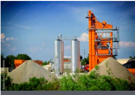
Asphalt mixing plants
